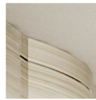
顶面造型 The top face shape
