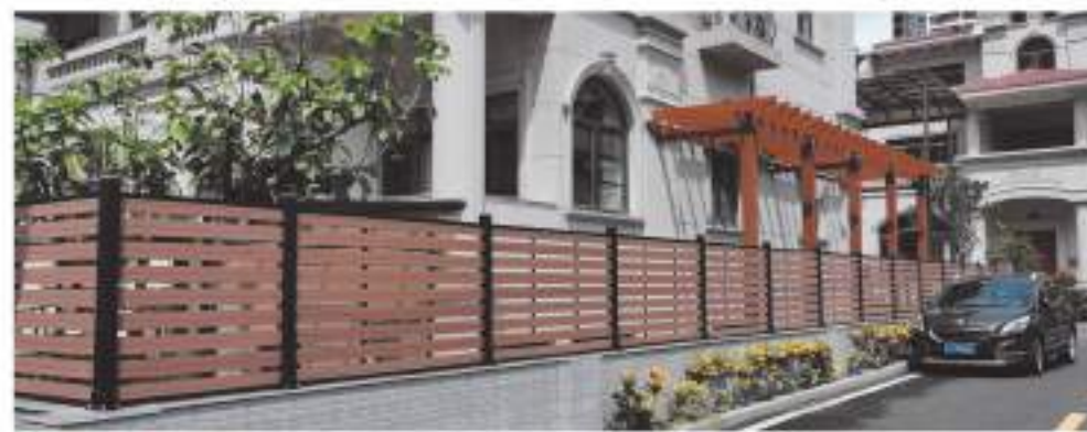
Jiangmen 1000meters Full-trellis Fence Project-2019
