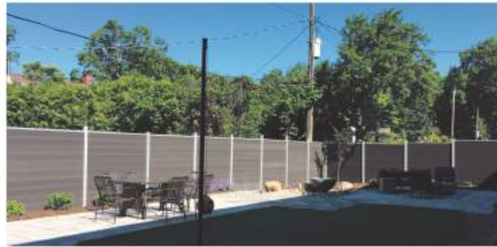
Canada 50meters Privacy Fence Project-2019
